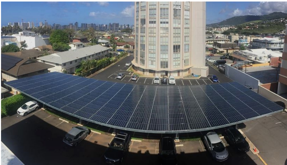
Building photovoltaic array over parking lot after March 2021 installation complete.
