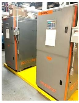
Replaced old hot water heaters with energy efficient on demand hot water heaters.
