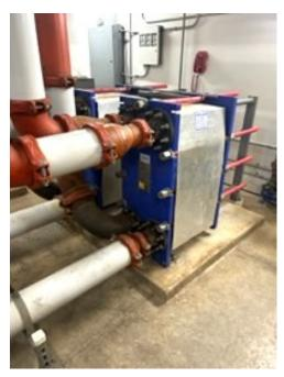
Replaced heat exchanger plates to help reduce energy loss for the condensing water.
